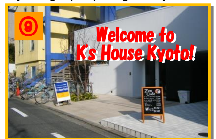
⑨ The reception for K's house is on the ground floor next to the entrance to Zen café. Enjoy your stay!!
